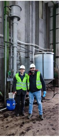
Similar to laboratory-scale batch experiments about 80% of phosphate was removed from LFD through struvite crystallization in the pilot-scale continuously fed, upflow reactor. The figure above shows the schematic of the pilot setup and a photograph taken during its operation.
