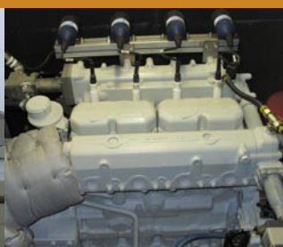
motor WKK: MAN 4 cilinder gasmotor
